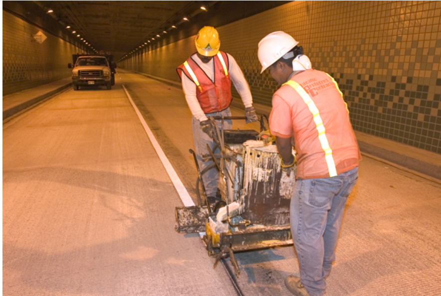
Figure 4: Restriping Wilson Tunnel, Likelike Highway, Oahu
