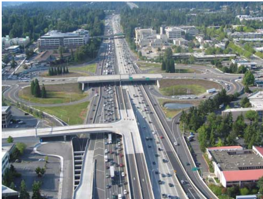
Figure 6: Washington Department of Transportation I-405 Corridor Program Project
